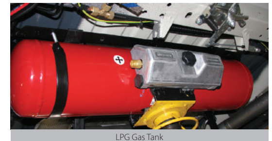
LPG Gas Tank
