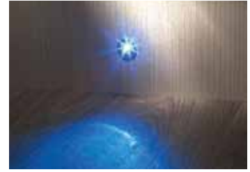
Built-in LED lighting at floor level to create a soft atmosphere and ensure that it's easy to move around at night in the living unit.
